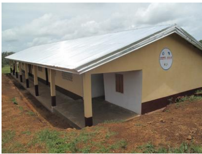
Completed classrooms at Rifem
